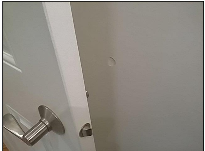
Wall damage at hall bath
