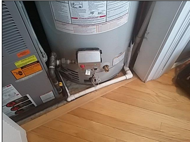
No drain pan at water heater
