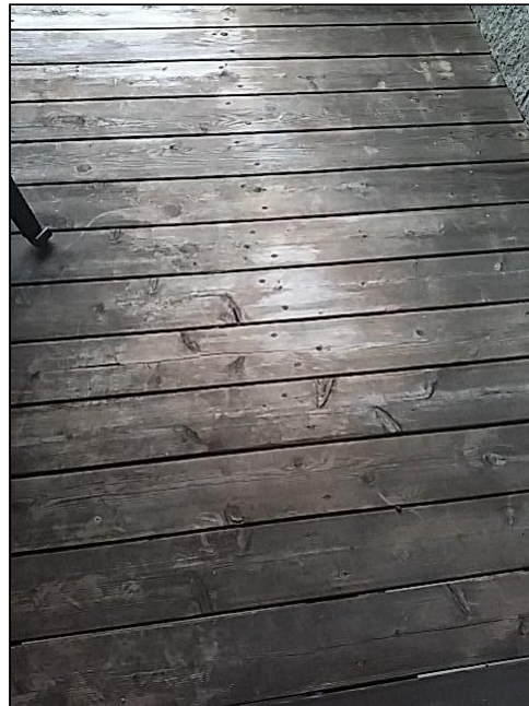
Weathered deck surface
