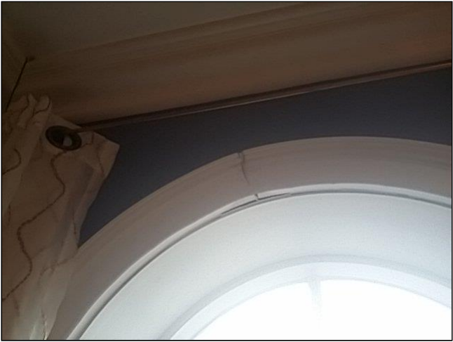
Moisture damage at wood trim
