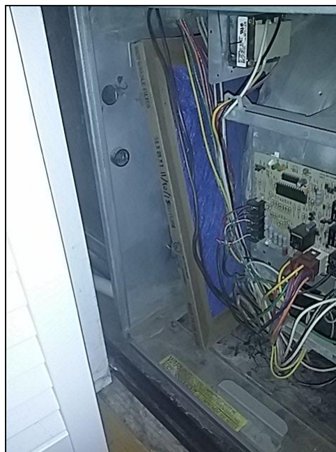
Filter not properly sealed in furnace
