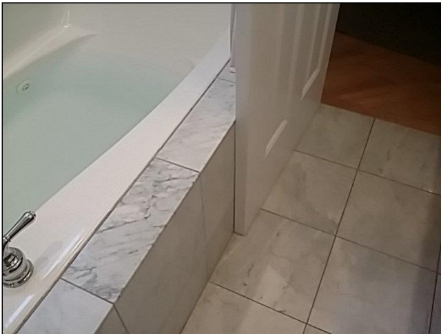
Master bath door strikes tub enclosure
