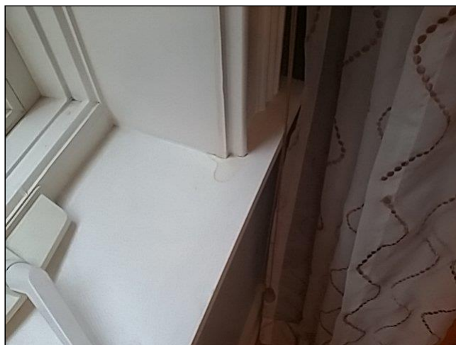
Water damage at living room window sill
