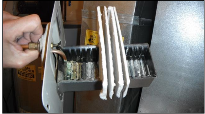
Typical humidifier interior
