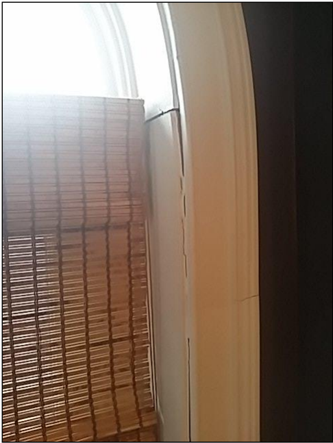
Moisture damage at wood trim
