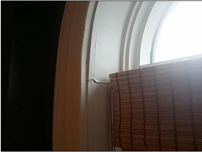
Moisture damage at wood trim
