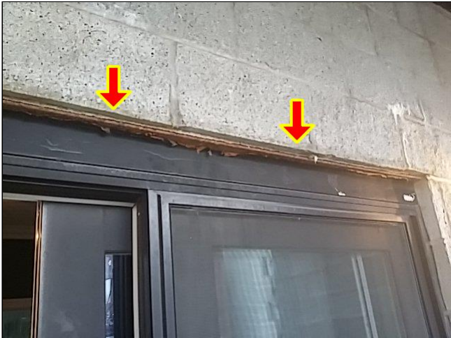
No visible flashing above doors
