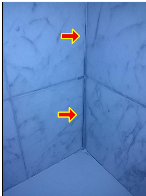
Repair cracked grout
