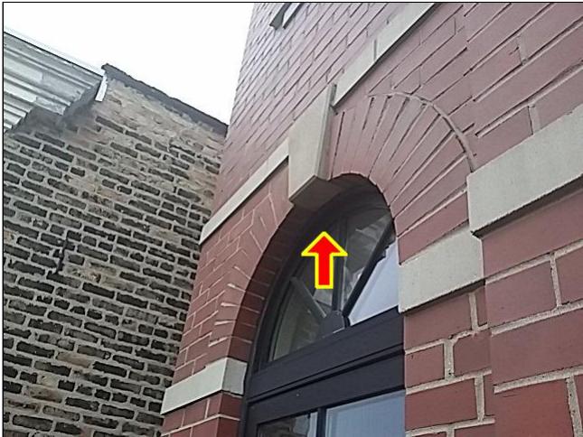
No visible flashing above windows
