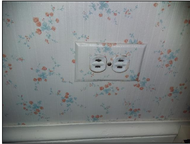
Replace 2 pronged outlets
