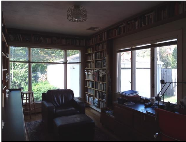
Windows will not open with control
