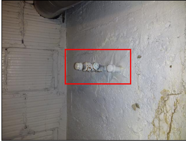
Pipes penetrating foundation wall
