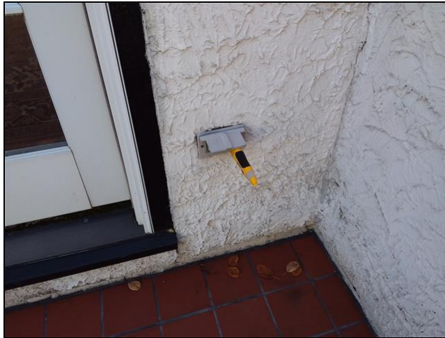
Outlet will not trip when tested
